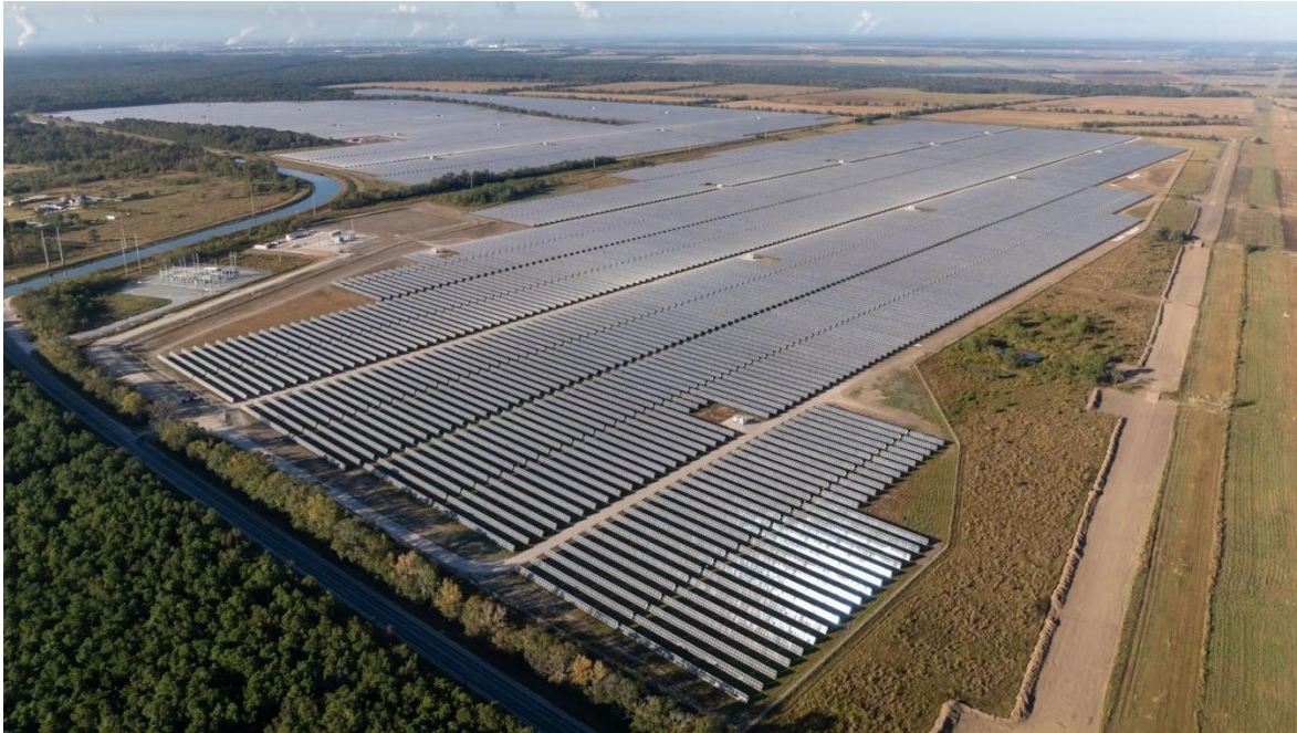
Actual 134MW system near Houston
