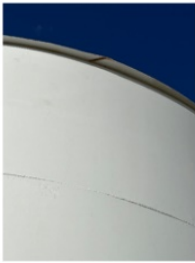
Exterior Wall Coatings
