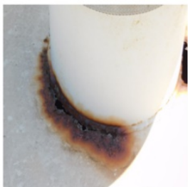
Exterior Roof Coating
