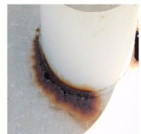
Exterior Roof Coating
