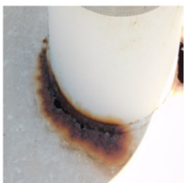
Exterior Roof Coating
