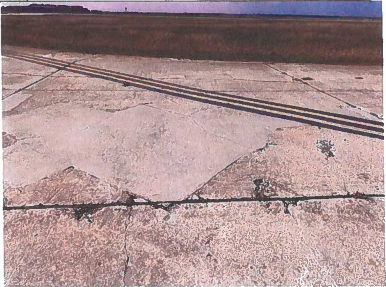
Figure 4 - Concrete patch completed along Taxiway A (Site Visit 10/24/22)
